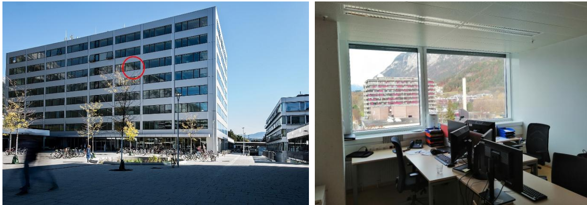
Figure 1: Office building of the Faculty of Engineering Sciences of the University of Innsbruck, Austria, with location of Room 518 marked with red circle (left; source original image: Universität Innsbruck/Birgit Pichler) and interior of the UIBK “Living Lab 518” three-person office (right).
